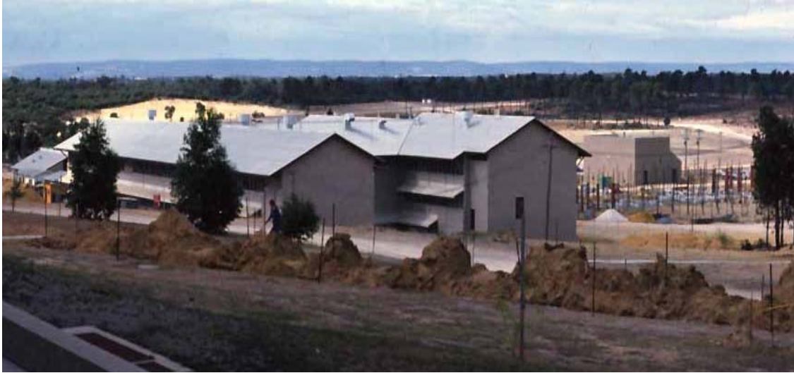
Fig 6: The building program was timed to correspond to the advance of the students through the course and was dominated initially by the building for the Division of Veterinary Biology (foreground). It contained staff offices and research facilities for the preclinical and paraclinical disciplines as well as teaching laboratories, museum and seminar facilities. A separate block containing necropsy rooms and holding areas was added slightly later.
